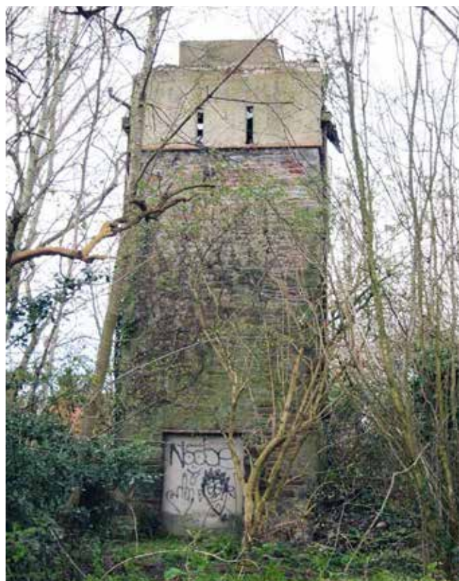
The engine house
